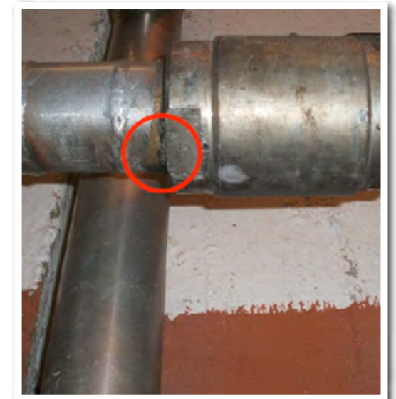
Leaks in water supply systems
