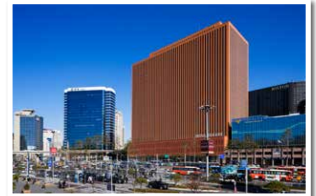
View after renovation
