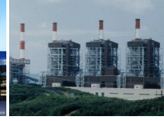
Boryeong Power Plant
