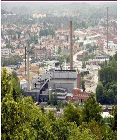
Energy storage (Boras, Sweden)
